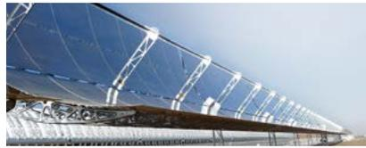
The Spanish company CIE EGAÑA is manufacturing support arms for the parabolic reflectors of a thermosolar plant under construction in Morocco. The new 125-megawatt plant will be one of the world's largest and the first thermosolar plant to be built in Morocco. Ruukki's metal-coated high-strength steel is being used to make the support structures.
