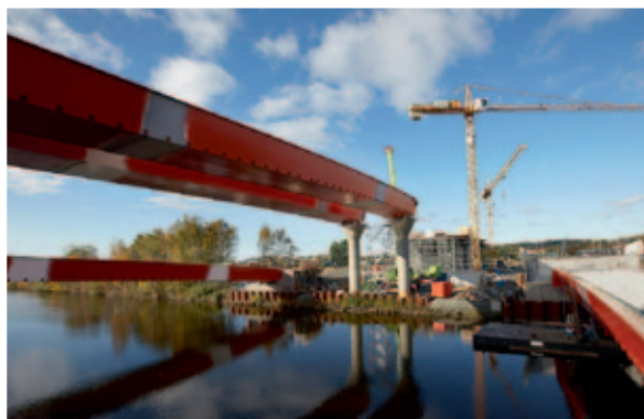
Ruukki's focus areas in infrastructure construction are transport infrastructure and harbour construction and building foundations. Partihallsförbindelsen link bridge interconnects the E45 motorway and E20 road.
