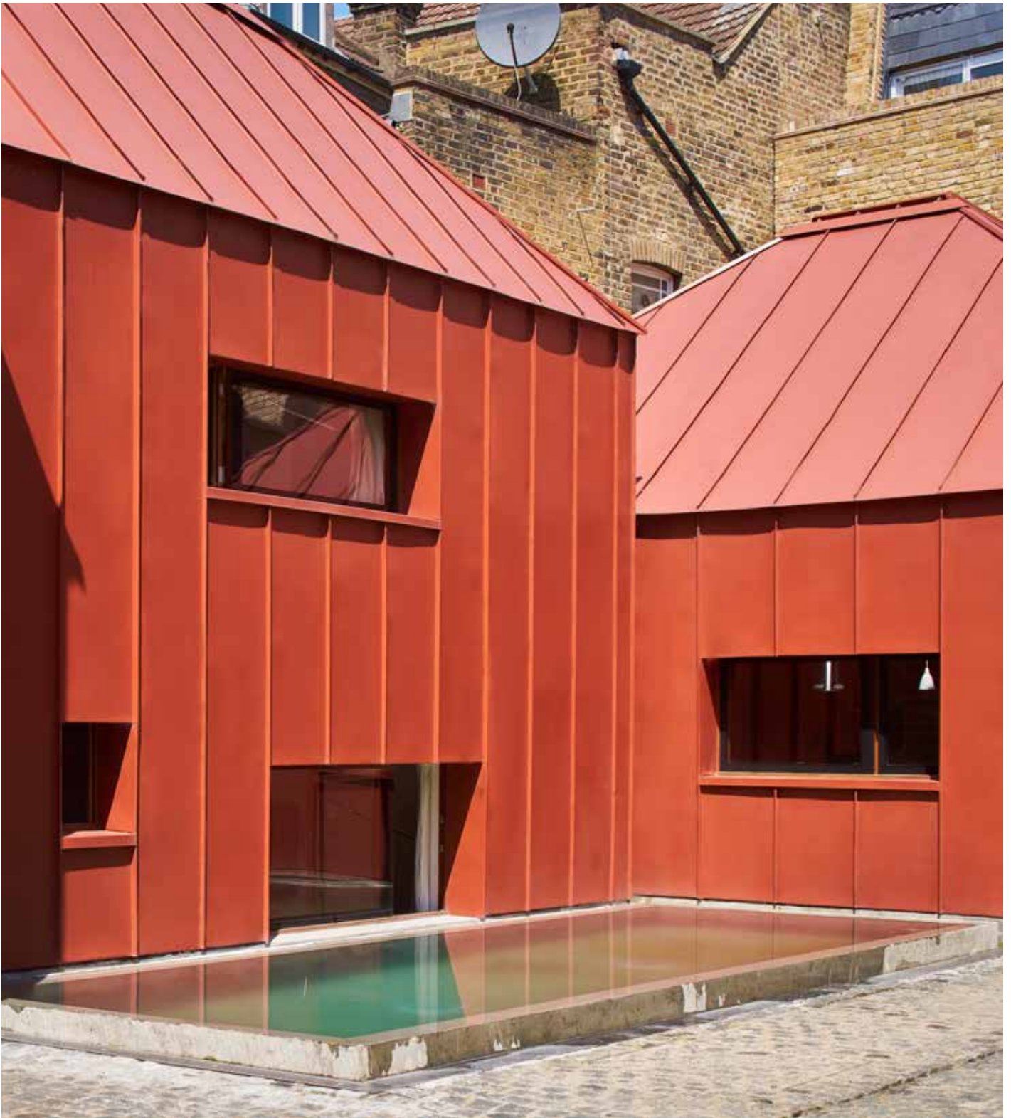
TIN HOUSE, LONDON, ENGLAND ARKITEKT: HENNING STUMMEL ARCHITECTS PRODUKT: GREENCOAT PLX PRO BT KULÖR: BRICK RED, RR7F2 / SS0742
