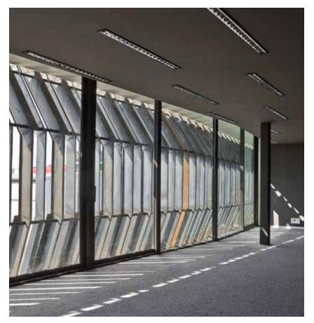
The front of the Audenasa Headquarters is made up of vertical COR-TEN® strips stretching the entire length of the building. Each strip is welded from three individual COR-TEN® sheets that have a 90 degrees bend at the edge.
