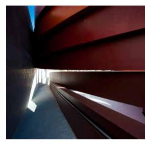
COR-TEN® steel was bent and welded to create the dynamic curved shapes that stretch around the Design Museum Holon's galleries and encircle the open public space in the center.
