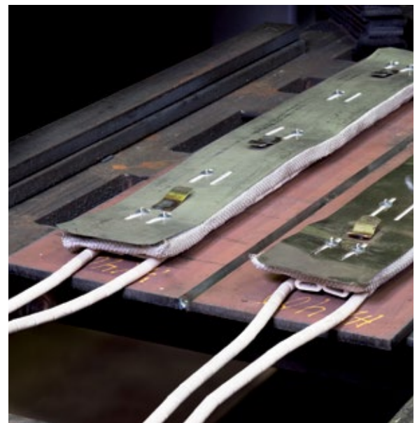
Figure 4 Using preheating blankets.
