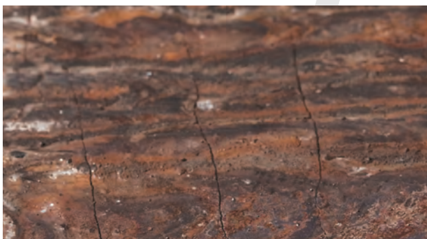
Fig. 20.8: Transverse cracks in a hardfacing layer.
