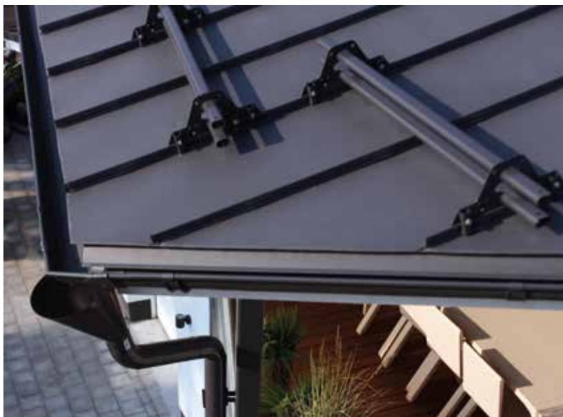
Figure 41. Snow guards manufactured from SSAB Form precision steel tubes.
