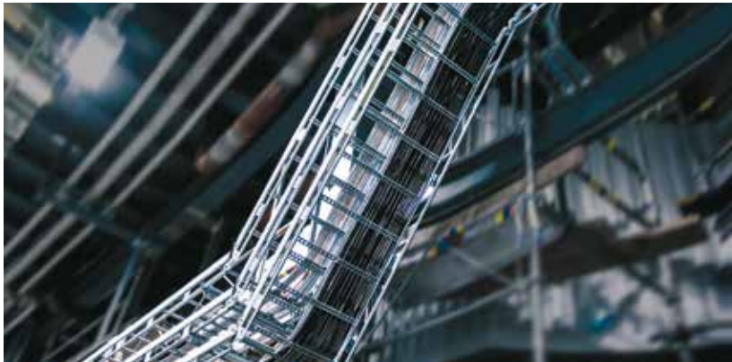
Figure 7. Cable ladder manufactured using a special tube profile. Courtesy of Meka Pro Oy.
