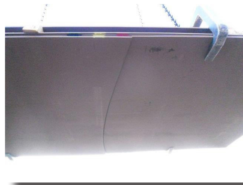
Example of a three-point lift with a crack as an result.
