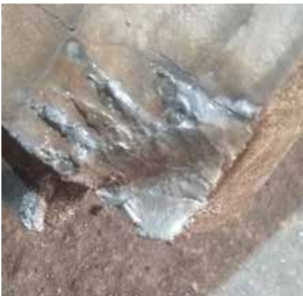
Chipped corner after cutting.
