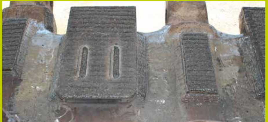
Plug filling of the oval hole when attaching a piece of Duroxite® plate to an excavator bucket.
