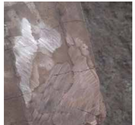
The repaired surface should be ground to become smooth and round.
